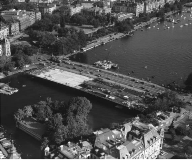
New bridge and temporary substructure in lake under construction
