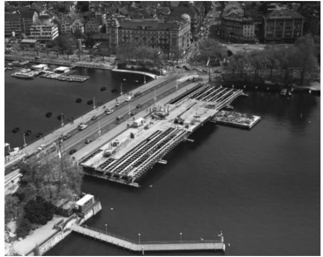
Demolishment of old bridge
