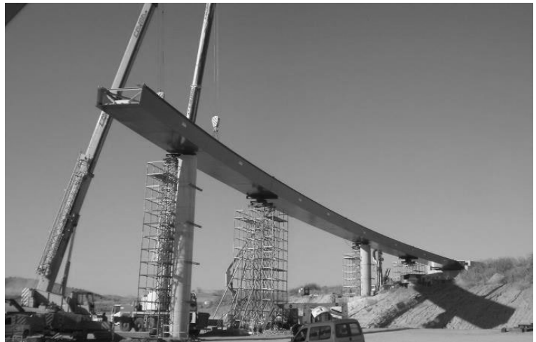
Erection of the steel member with temporary supports
