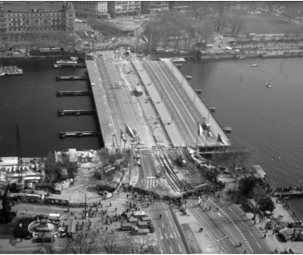
Two bridges travelling towards the lake
