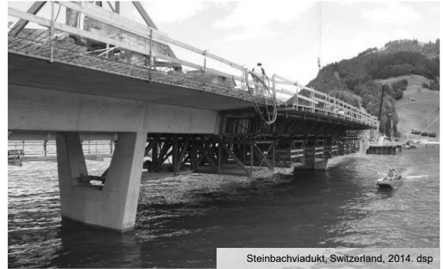
Steinbachviadukt, Switzerland, 2014. dsp
