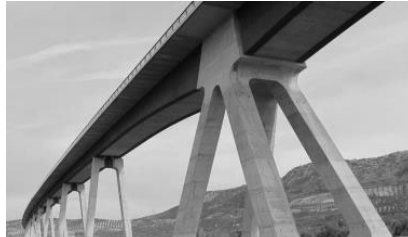
Archidona viaduct, Spain, 2012. IDEAM
