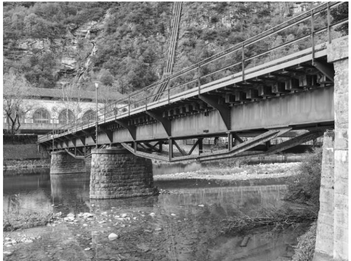
Example: Steel superstructure on stone masonry piers, concrete abutments (Ticino Bridge Atel, photo © Georg Aerni)
