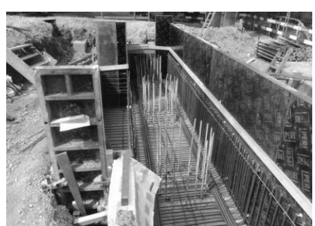
Pile cap formwork
