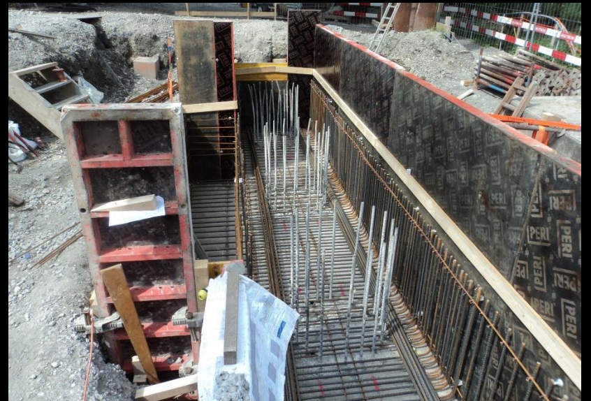
Pile cap formwork
