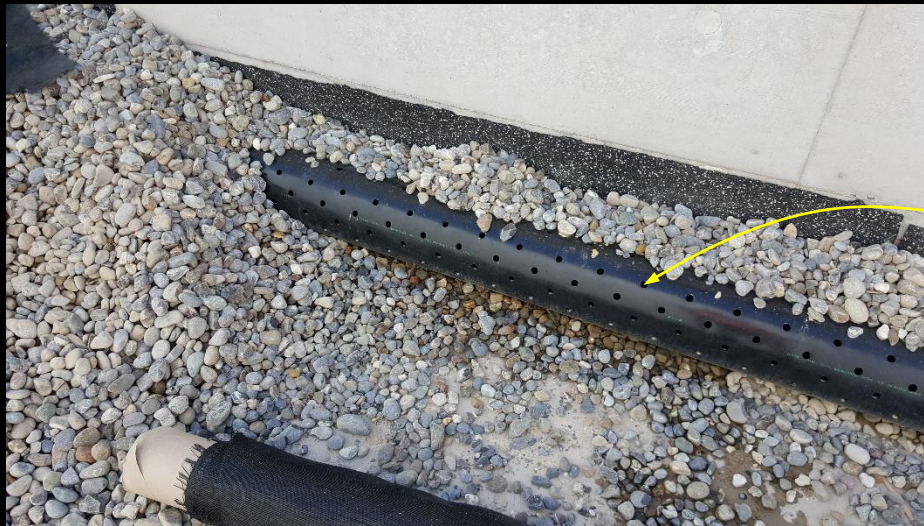
Seepage pipe at abutment base
