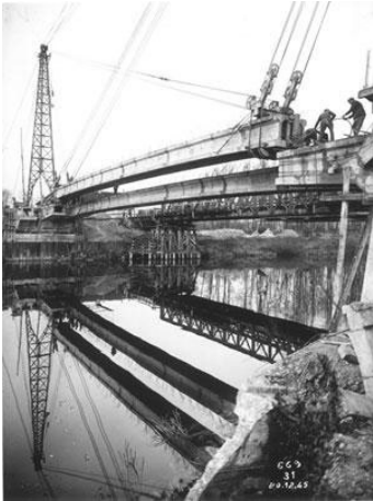
Marnebrücke Luzancy (1941-46) Eugène Freyssinet
