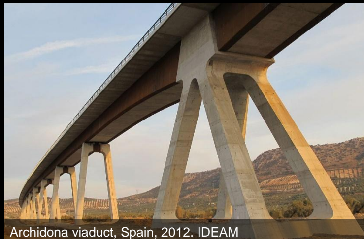
Archidona viaduct, Spain, 2012. IDEAM
