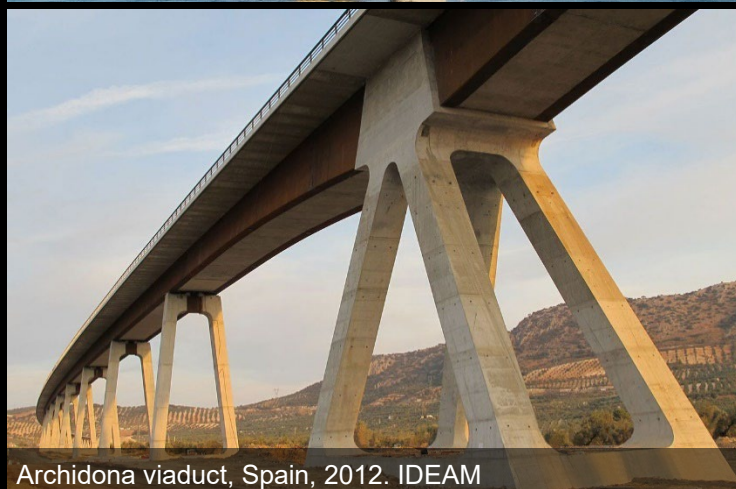
Archidona viaduct, Spain, 2012. IDEAM
