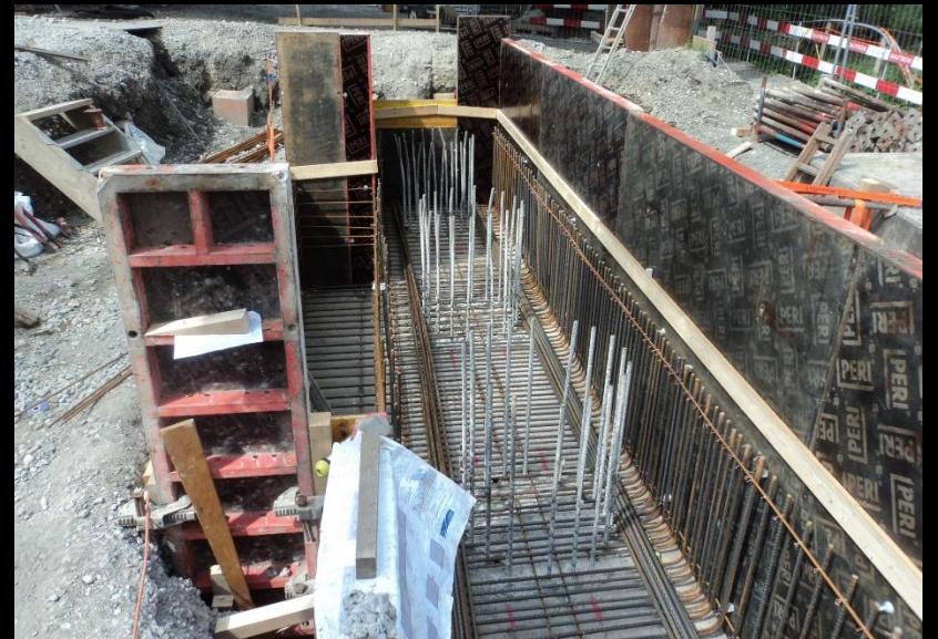
Pile cap formwork
