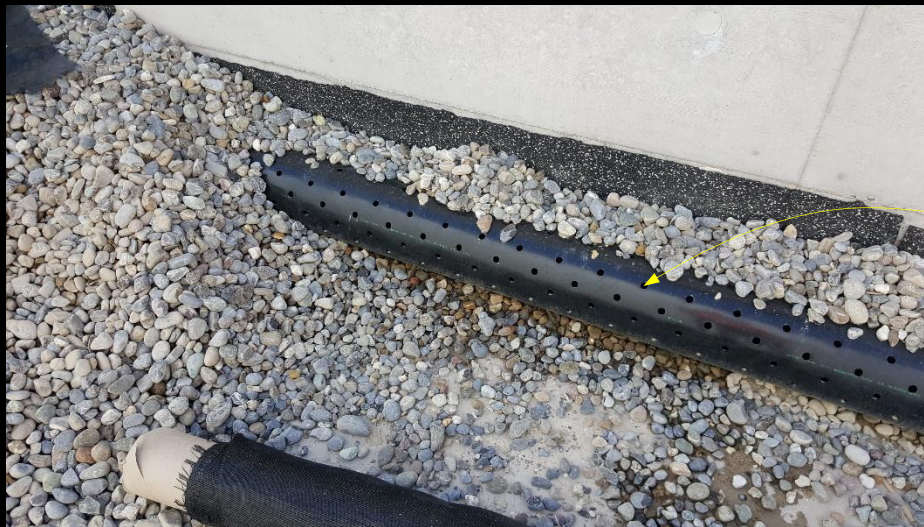
Seepage pipe at abutment base
