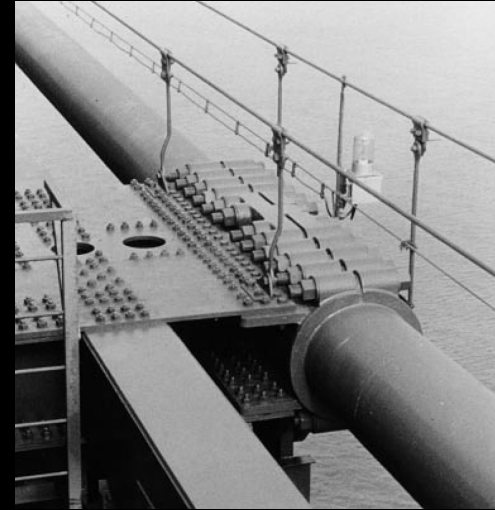
Central clamps at midspan: Examples
