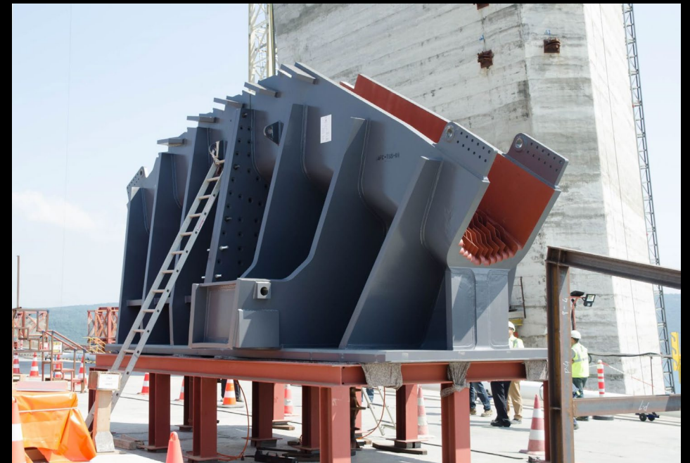
Tower saddle of Third Bosphorus Bridge
