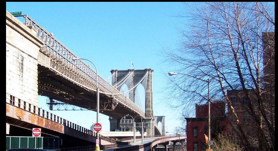
Brooklyn bridge: Extreme side spans, l_s / l_m = 0.59
