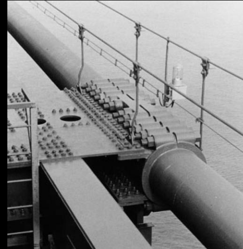
Central clamps at midspan: Examples
