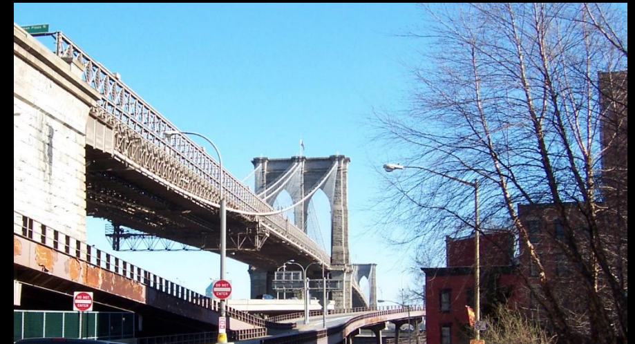
Brooklyn bridge: Extreme side spans, l_s / l_m = 0.59
