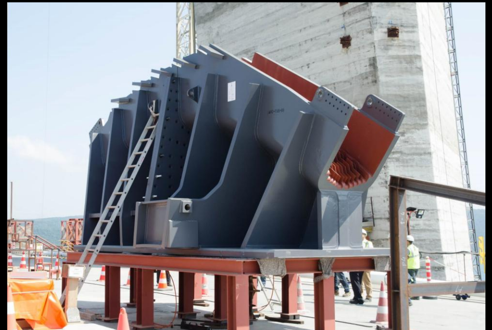
Tower saddle of Third Bosphorus Bridge
