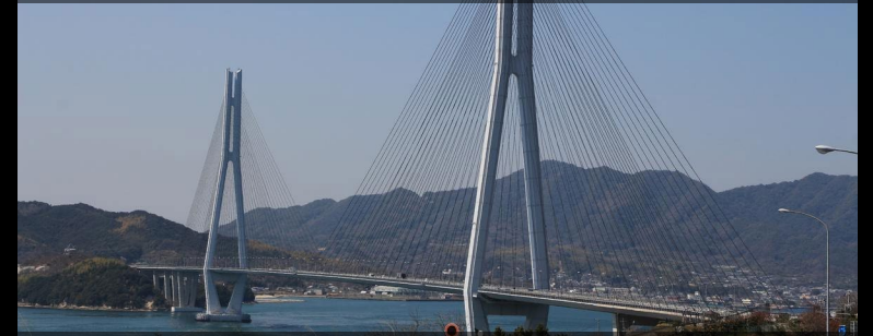
Tatarabashi Bridge, Japan, 1999. Honshu-Shikoku Bridge Authority
