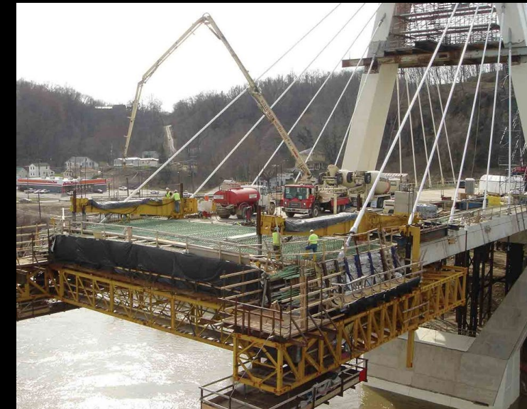
Sidney Lanier Bridge, Brunswick, GA, USA, 2003. TYLI
