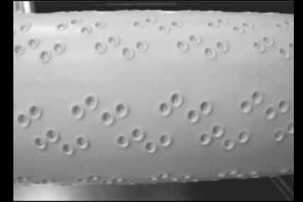
Rain-wind induced vibrations of stay cables (Franjo Tuđman Bridge, Dubrovnik)
