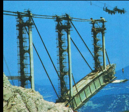
assembly of arch basic section (cantilevered part)
