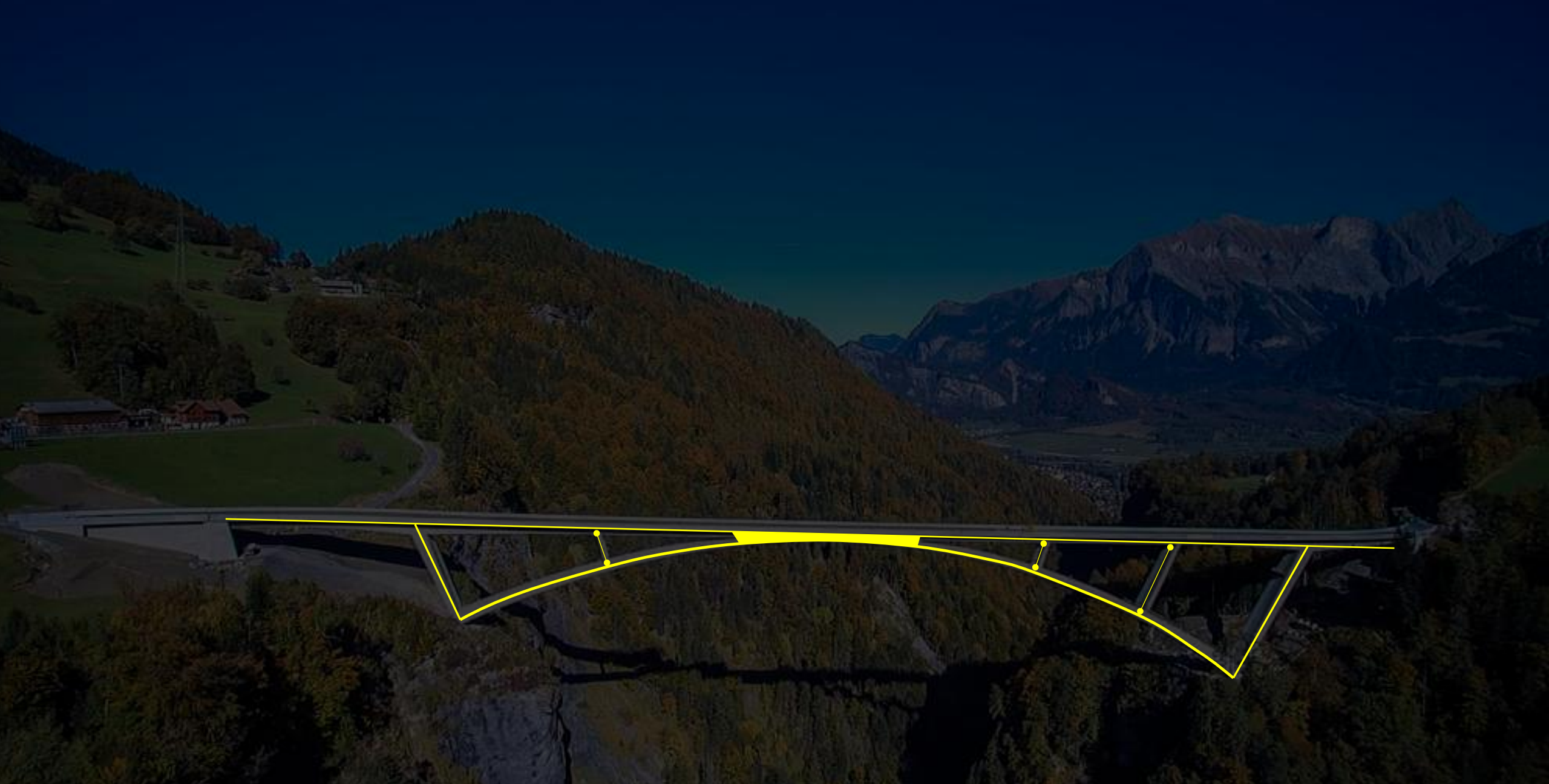
Tamina bridge, Switzerland, 2016. Leonhardt, Andrä und Partner
