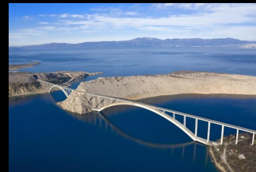
Krk Bridge, Croatia
