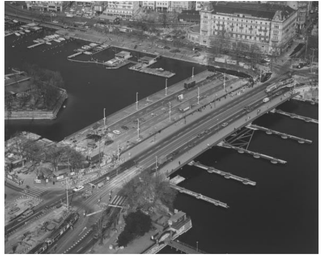
New bridge and launching tracks (almost) ready for launching
