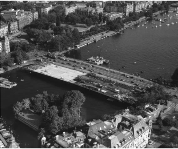
New bridge and temporary substructure in lake under construction
