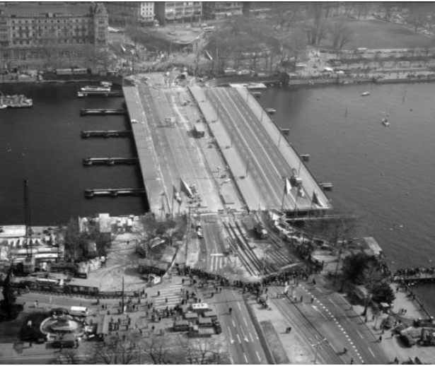
Two bridges travelling towards the lake
