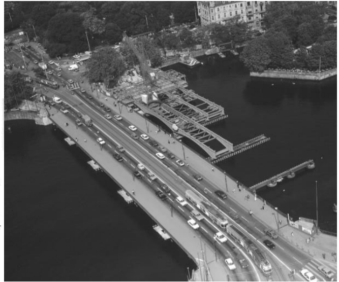
New bridge under construction (downstream of old bridge)
