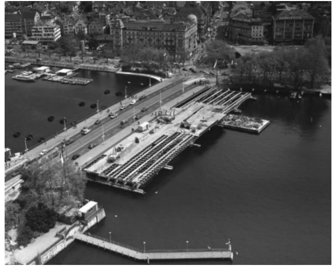
Demolishment of old bridge
