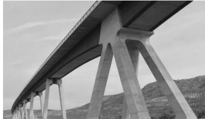
Archidona viaduct, Spain, 2012. IDEAM
