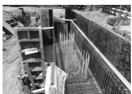
Pile cap formwork
