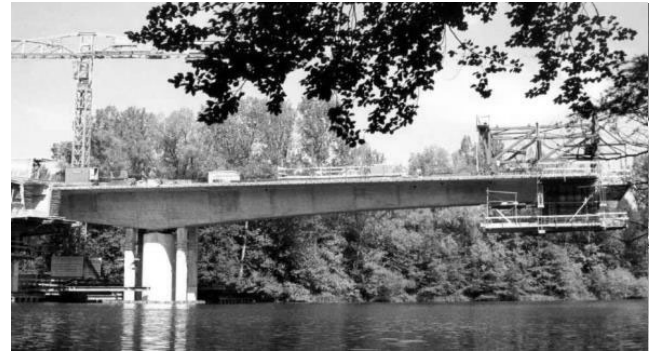
Balanced cantilevering from pier with bearings (temporary supports)
