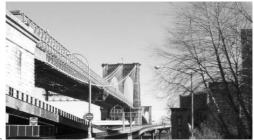
Brooklyn bridge: Extreme side spans, l_s / l_m = 0.59
