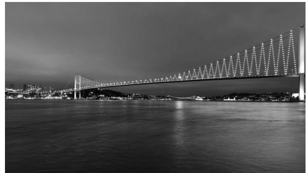
Suspension bridges with Inclined hangers and hanger network
