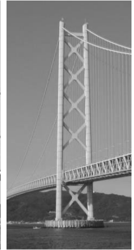
Diagonally braced tower: Akashi-Kaikyo bridge
