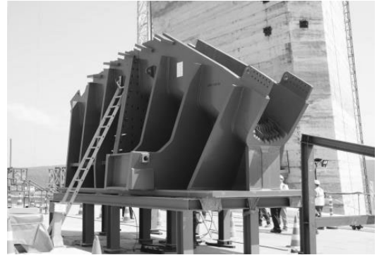
Tower saddle of Third Bosphorus Bridge
