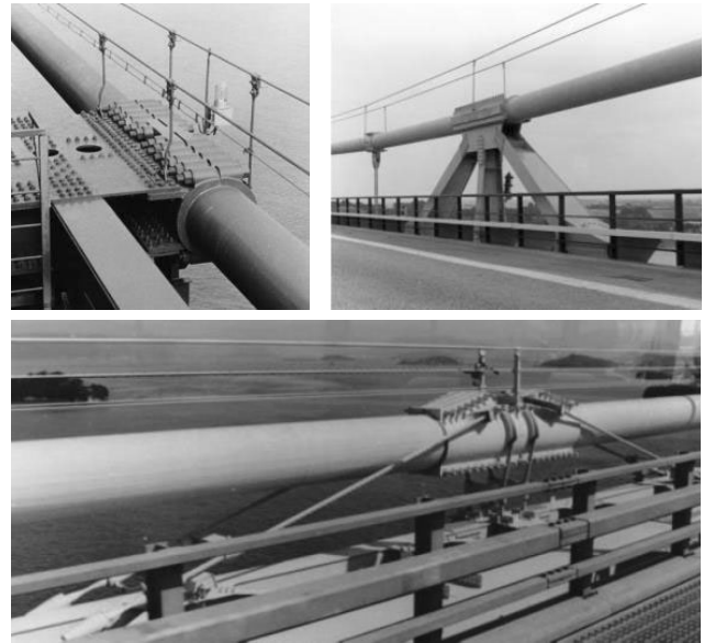
Central clamps at midspan: Examples
