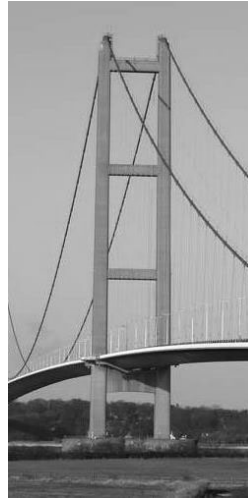
Portal-type tower: Humber Bridge
