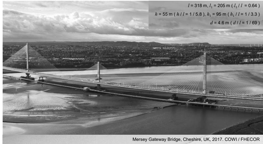
Finally, in the case of the Mersey Gateway Bridge, the spans are proportioned so that the interior tower is shorter than the ones stabilised by backstays, thus reducing the tributary span for the interior tower and its slenderness (compared to the exterior towers).
