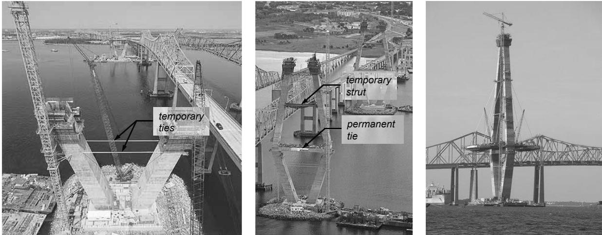
The inclined legs of the lower half of the diamond are erected in lifts. At a certain height, to control the bending moments at the base of the legs, a temporary tie is installed (pictured left).
