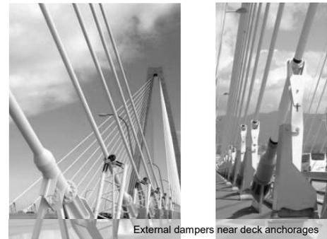
Note that the parallel strand stay cables most commonly used in modern cable-stayed bridges have a relatively low density. As a result they feature a relatively low Scruton number,  $Sc$ :
