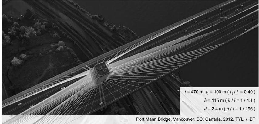
Multiple inclined plane arrangements combined with a single tower can help to minimise the foundation footprint. The Port Mann Bridge had the widest deck in the world when it opened, with 10 lanes of traffic.
