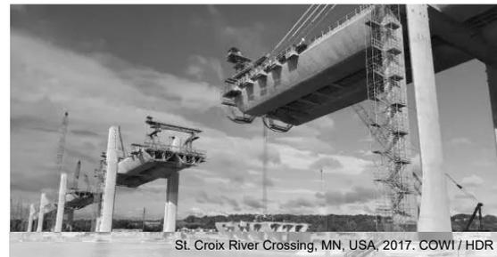
Successful stay installation based on stay length relies on accurate surveying and knowledge of the forces acting on the girder (construction equipment loads) during installation.
