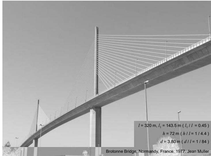
Single plane arrangements result in clean aesthetics, are possible for narrow to medium width decks, and are combined with box girders (torsional rigidity provided by the closed section is required to resist eccentric loading). They are typically supported by single towers (pictured). Inverted “Y” towers are also common (see behind).
