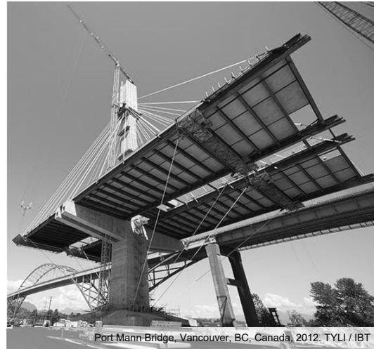
Composite girder systems typically feature precast deck slabs that have cured sufficiently to allow the majority of shrinkage strains to occur unrestrained.
