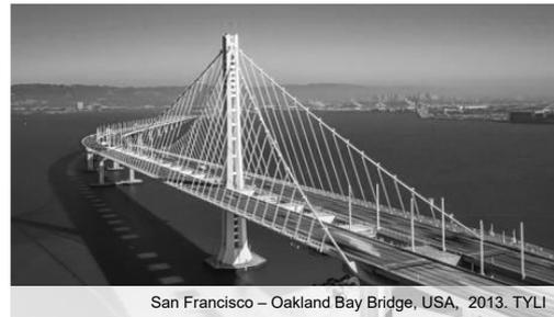
The main span of the new San Francisco – Oakland Bay Bridge (pictured bottom right) is an example where the owner (with public input) opted for a self-anchored suspension bridge to match the aesthetics of the neighbouring existing Bay Bridge and the Golden Gate Bridge (both suspension bridges built in the 1930's). A cable-stayed bridge (rendered top right) would have been much more economical.
