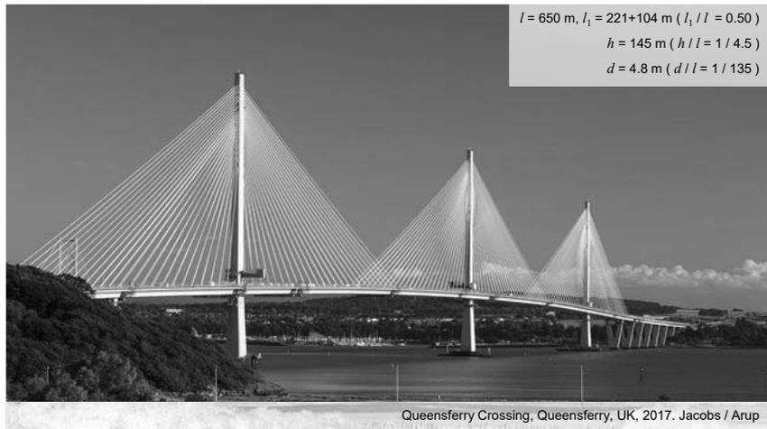
In the case of the Queensferry Crossing, the structure is stiffened by overlapping the main span stay cables. One disadvantage of this approach is that a wider bridge deck is required to accommodate the anchorages of the overlapping stay cables.
