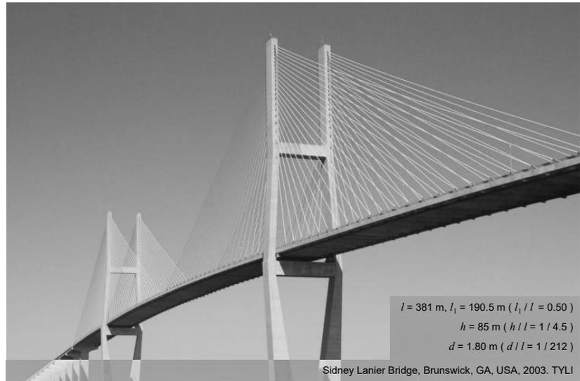
Two vertical planes arrangements are typically combined with open cross-section superstructures. Box girders are also sometimes used but are less convincing in appearance, unless slender and streamlined. They are typically combined with “H” towers (pictured).
