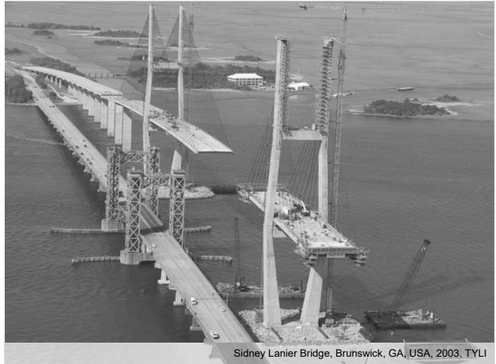
Flexible girder systems originated in Germany. Emphasis is placed on the axial loading of the stay cables and away from the bending strength of the girder (axial loading is more efficient than bending).
