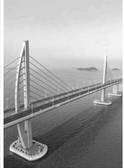
As in the case of girder bridges, the substructure elements (tower in this case) offer the opportunity to enhance the aesthetic appearance of cable-stayed bridges, often with minimal impact on total construction cost. However, it is also possible to result in structures that appear contrived where the form does not follow function.
