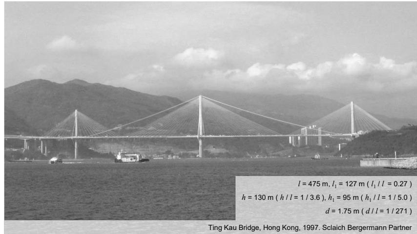
A unique approach was used to stabilise the interior tower of the Ting Kau Bridge, with the use of special-purpose stay cables that connect the top of the interior tower to the point where the superstructure intersects with the exterior towers.
