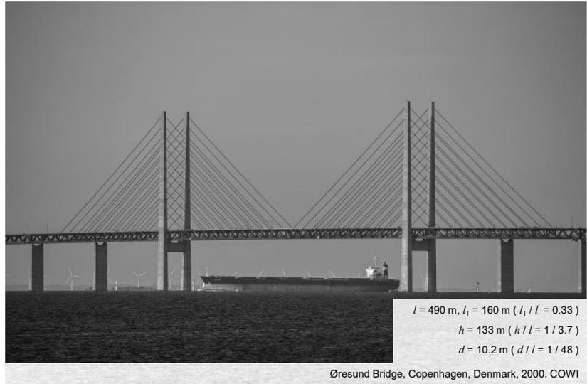
The harp arrangement is favoured by architects due to the clean aesthetics. However, it is the least economical system because all stay cables have a relatively flat inclination. In addition, the shorter lower stays are significantly stiffer compared to the longer upper stays and can attract very high forces, e.g. in the case of high seismic forces (in the longitudinal direction) combined with a floating deck at the tower.
