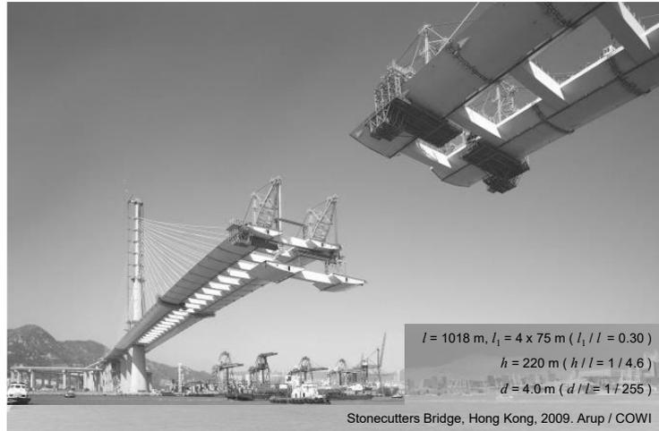
Typically used for spans longer than 600 m, where savings in weight and a streamlined cross-section is required.
