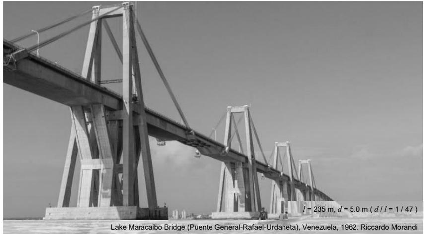
Span arrangements that include more than three spans, and correspondingly more than two towers, are classified as multi span. The interior spans and towers lack the advantage of being stabilised by backstays and anchor piers. Therefore, alternative measures must be taken to stiffen the structure. The approach taken in the Lake Maracaibo Bridge was to use very stiff towers that can resist unbalanced loading of the interior spans.
