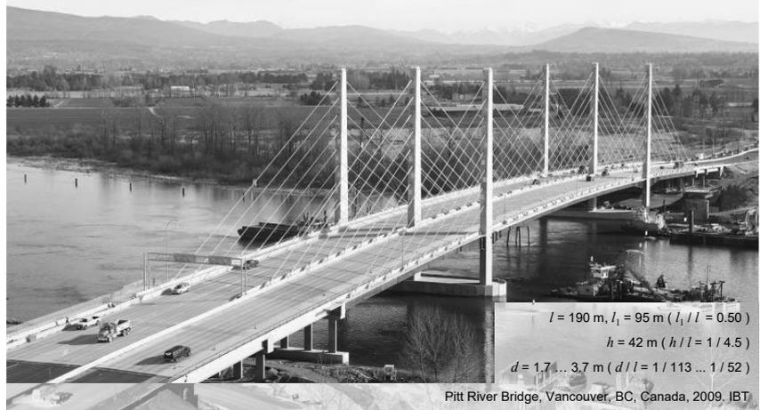
For very wide decks, it becomes more efficient to add a plane of cables, rather than relying on the deck to span transversely between two cable planes. Harp cable arrangements (pictured) are often preferred in the case of multiple cable planes to improve transparency from every viewing angle.
