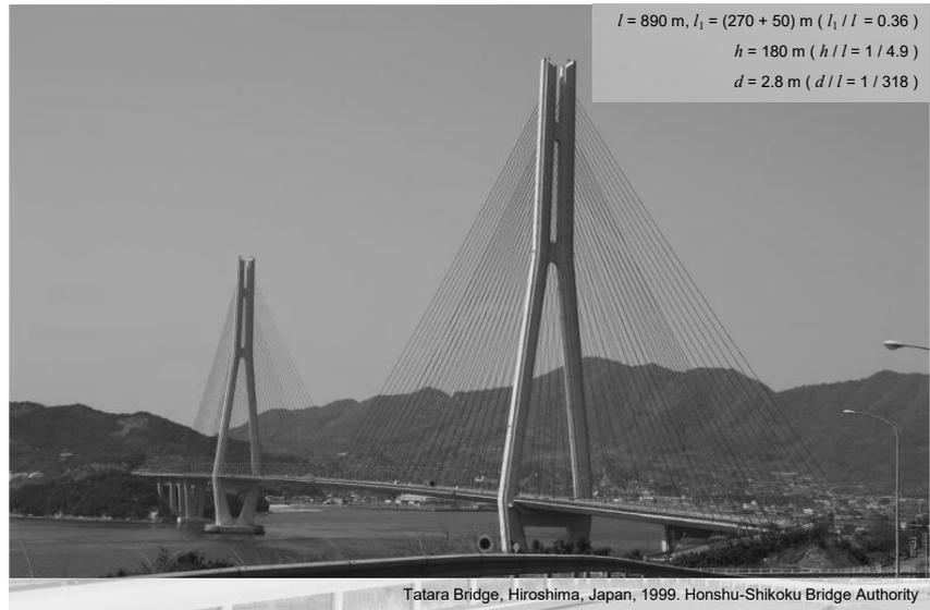
Inclined planes are used in combination with “A”, Diamond or Inverted “Y” towers (see behind) in order to improve the aerodynamic performance of very long spans.
