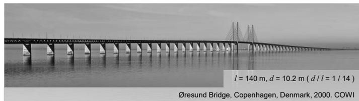
Commonly used in the case of railway bridges and/or where double-deck systems are employed.
