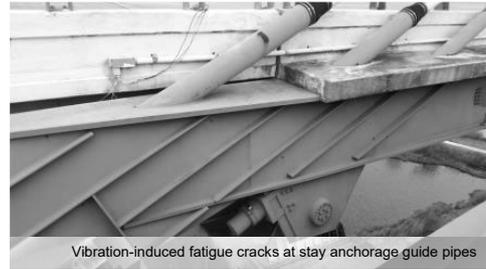
Vibration-induced fatigue cracks at stay anchorage guide pipes
