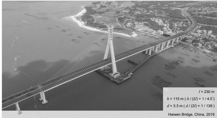
The symmetric two-span configuration is not very common, but can be an appropriate solution to meet specific site constraints. It is generally advantageous to opt for an asymmetric span layout, as this results in a stiffer structure (see behind).
