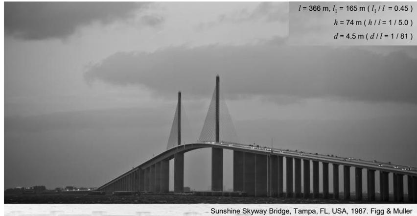
Single towers are the simplest form of tower, are typically supporting a single plane of cables, but can also support two or more inclined planes.
