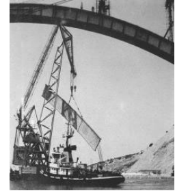
hoisting of outer arch ribs
