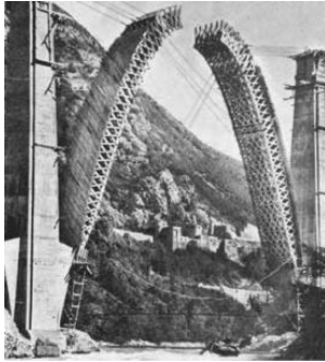
Rotation of centering for the Longeray arch bridge
