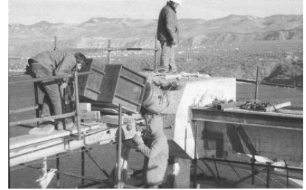
deck erection (precast girders)
