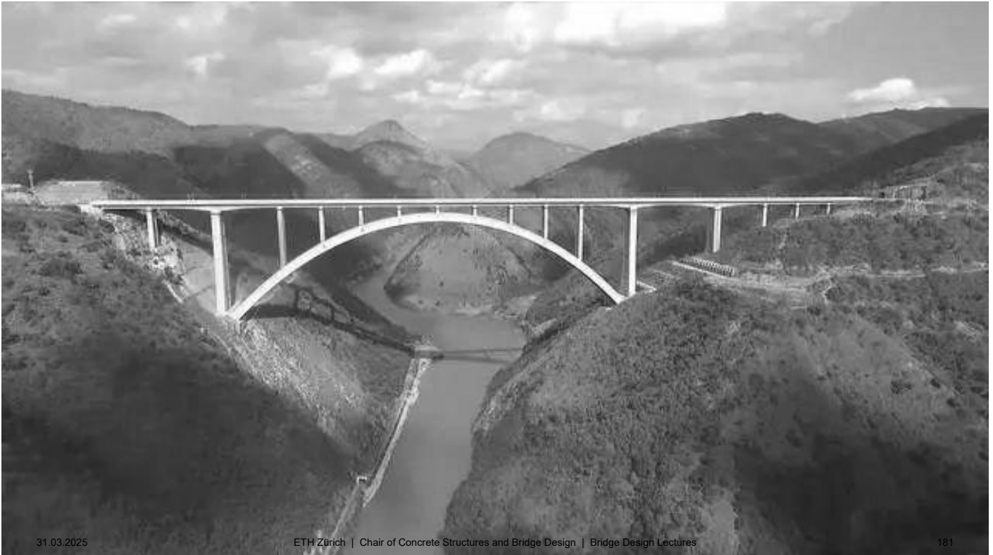
Yunnan–Guangxi Railway Nanpan River Bridge (aka Nanpanjiang Railway Bridge Qiubei), CFST reinforced concrete deck arch bridge, span 416 m, f/L = 1/4.2 , total length 852 m.
