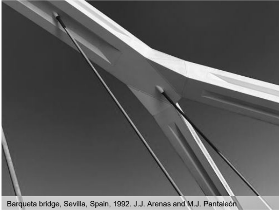
Barqueta bridge, Sevilla, Spain, 1992. J.J. Arenas and M.J. Pantaleón
