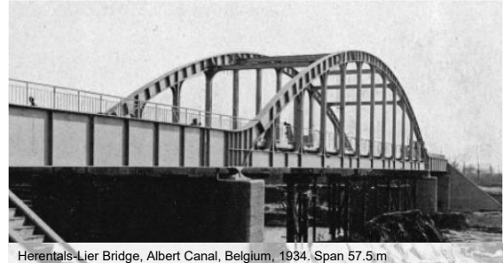
Herentals-Lier Bridge, Albert Canal, Belgium, 1934. Span 57.5 m
