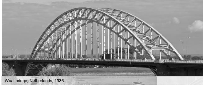
Waal bridge, Netherlands, 1936.
