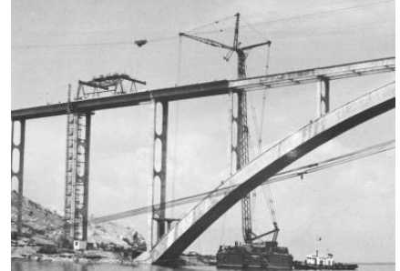
deck erection (precast girders)
