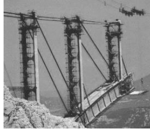
assembly of arch basic section (cantilevered part)
