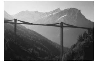
Gantner Bridge, Switzerland
