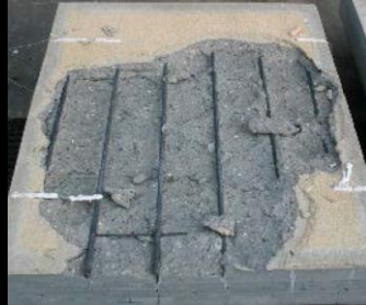
Explosive spalling after 119 min of fire exposure d_p = 10 mm
