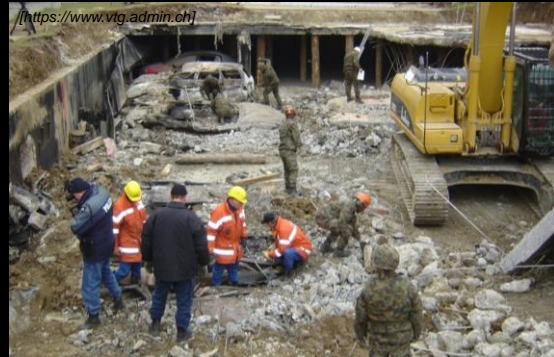
Fire in underground car parking, Gretzenbach (2004)
