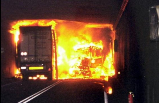
Fire in St. Gotthard tunnel (2001)
