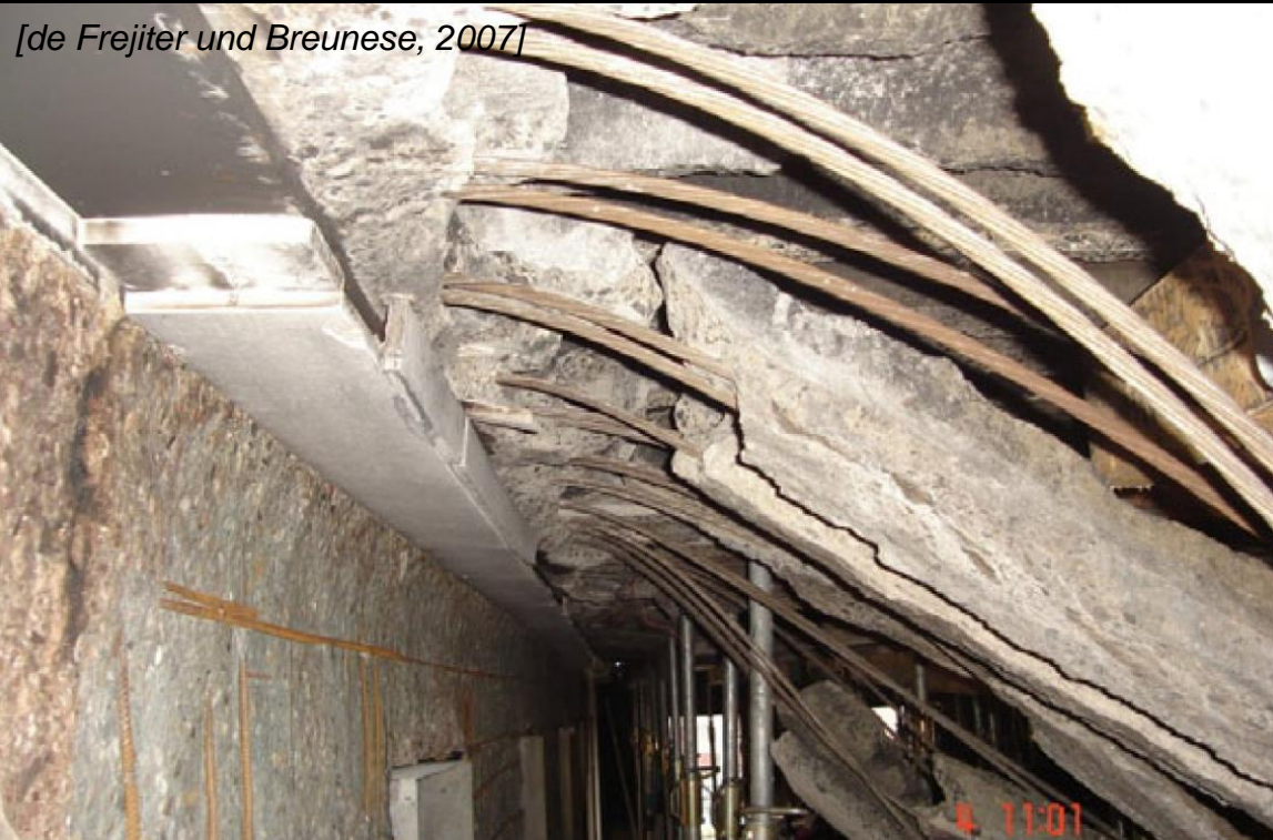
Fire in underground car parking, Rotterdam (2007)
