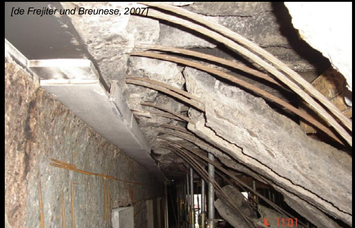
Fire in underground parking, Rotterdam (2007)
