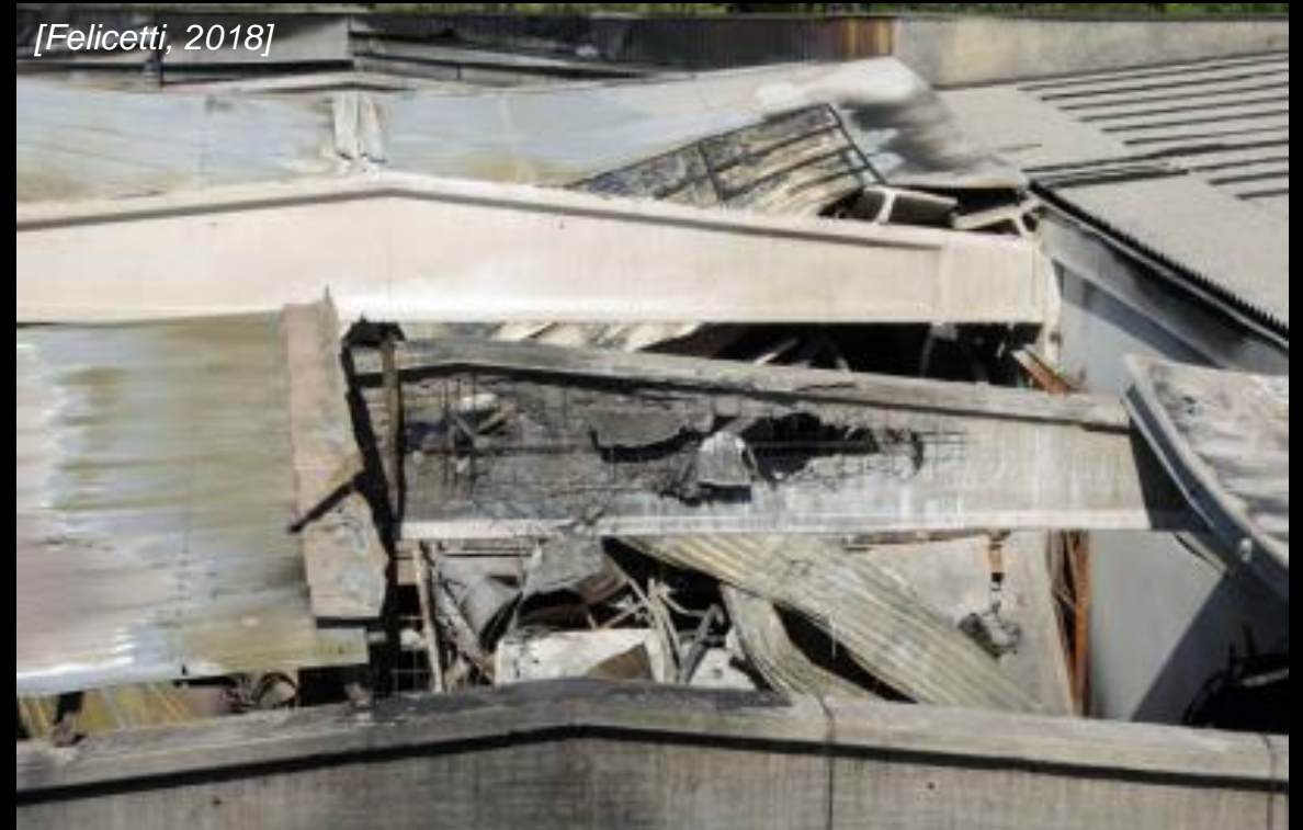
Fire in warehouse, near Milano (2018)
