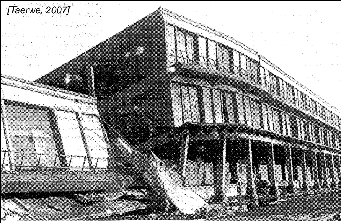
Fire in warehouse, Gent (1974)
