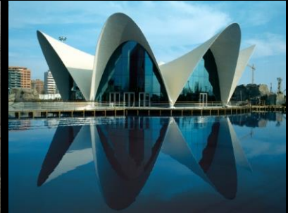
Thin shell structures (with conventional reinforcement)
