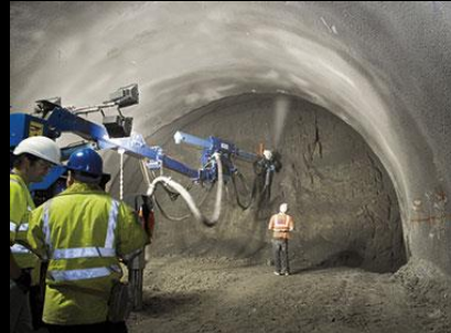
Shotcrete for tunnel lining
