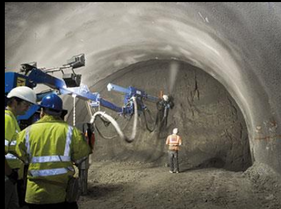
Shotcrete for tunnel lining
