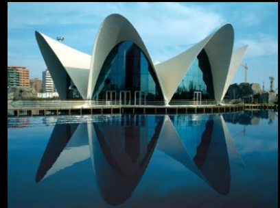
Thin shell structures (with conventional reinforcement)
