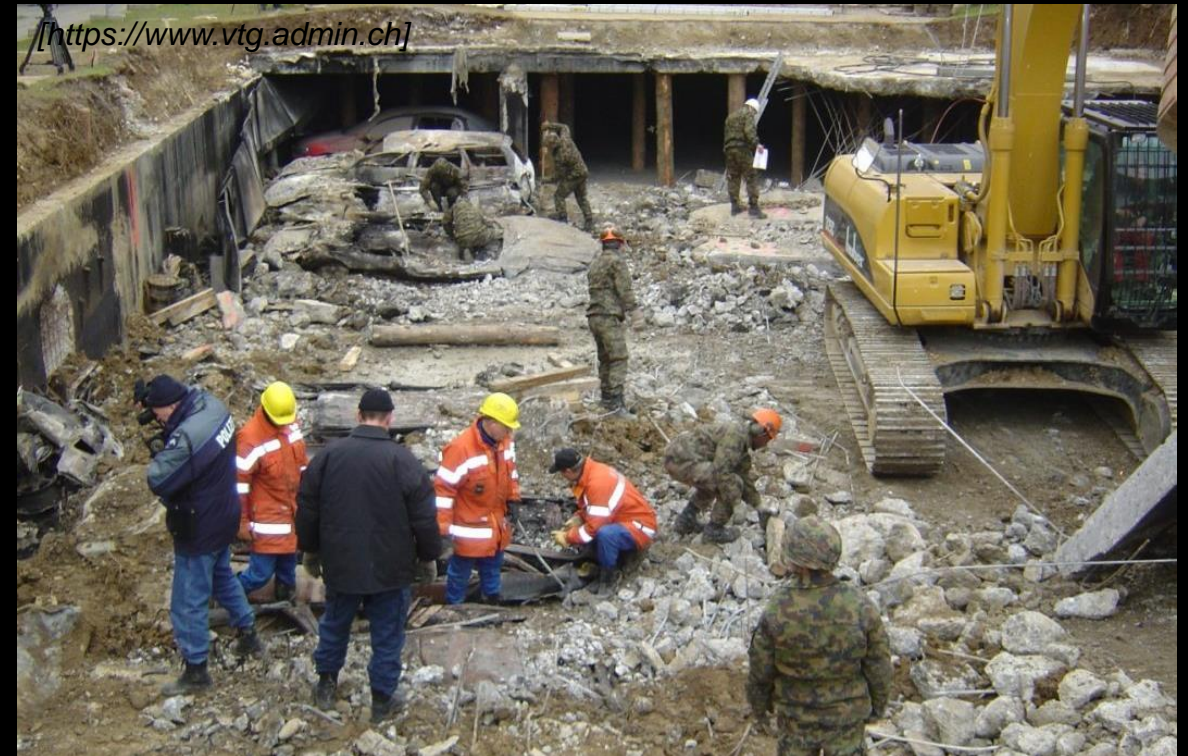
Fire in underground car parking, Gretzenbach (2004)
