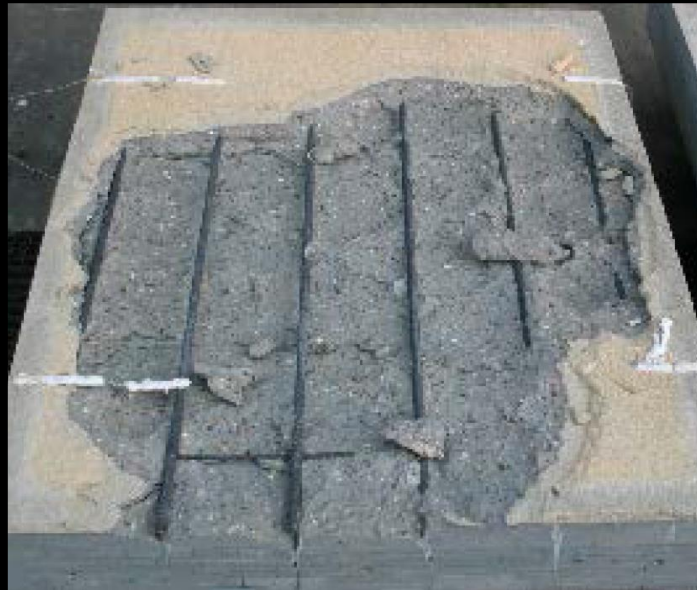
Explosive spalling after 119 min of fire exposure d_p = 10 mm
