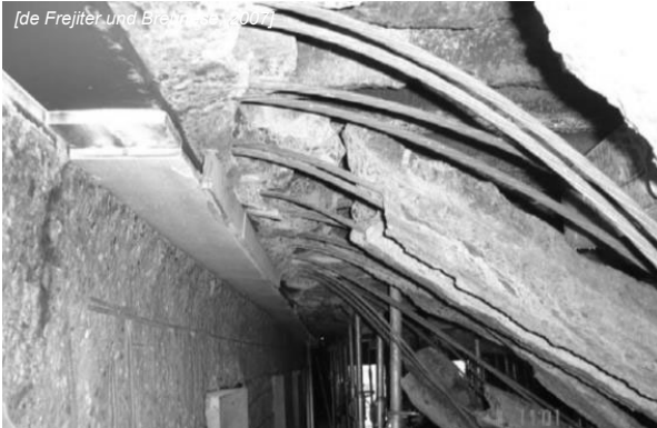
Fire in underground car parking, Rotterdam (2007)
