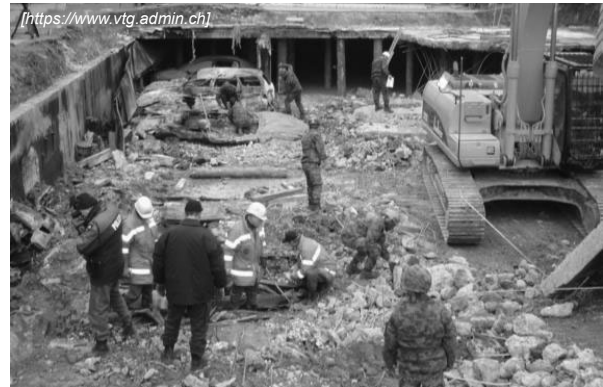
Fire in underground car parking, Gretzenbach (2004)
