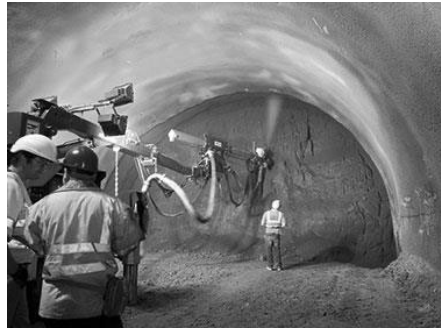
Shotcrete for tunnel lining
