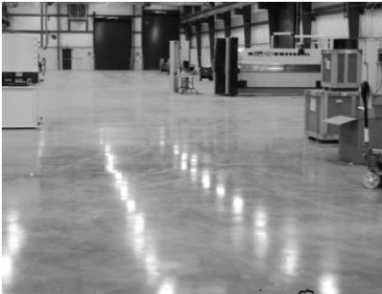
Slab on grade
