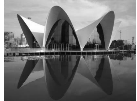
Thin shell structures (with conventional reinforcement)
