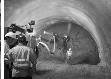
Shotcrete for tunnel lining
