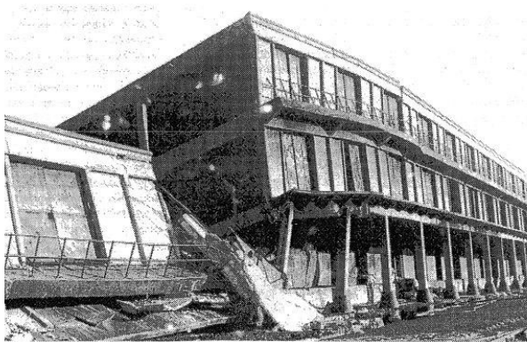
Fire in warehouse, Gent (1974)
