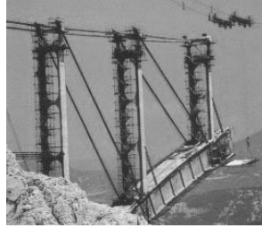
assembly of arch basic section (cantilevered part)
