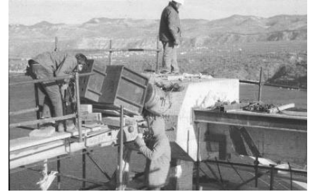
deck erection (precast girders)
