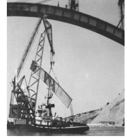
hoisting of outer arch ribs
