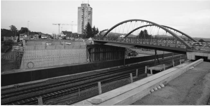
SBB Bridge Oftringen, Switzerland, 2018, Fürst Laffranchi Ingenieure GmbH / IUB Engineering
