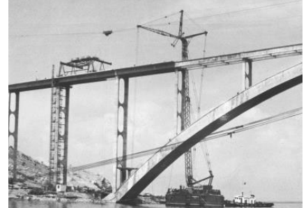
deck erection (precast girders)
